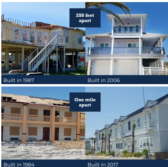
Figure 1. Two examples of damage to older versus newer construction after Hurricane Harvey.
