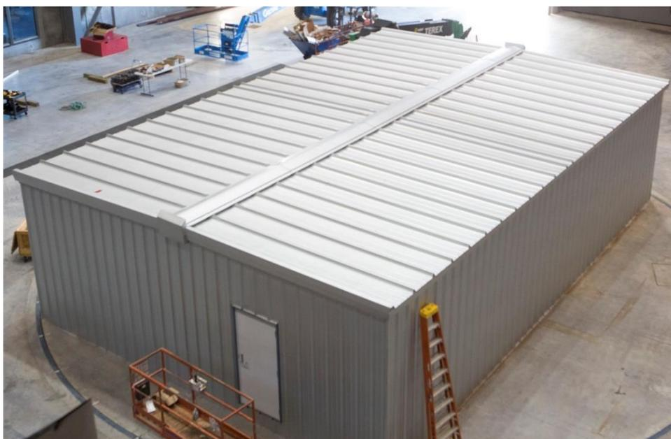
Figure 1. Photograph of the completed test building using a sculpted eave trim.
