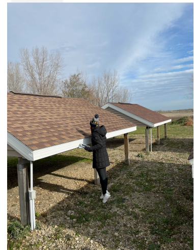
Figure 2. IBHS staff conduct annual visual inspections of each specimen.
