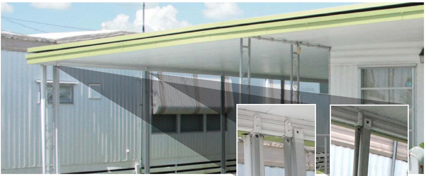
Figure 18. Posts added next to existing decorative post and pipe posts.
