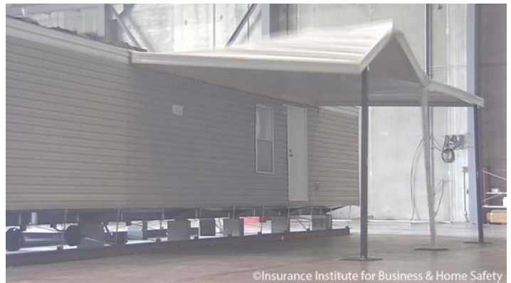
Figure 6. Buckling of beams supporting roof edge.
