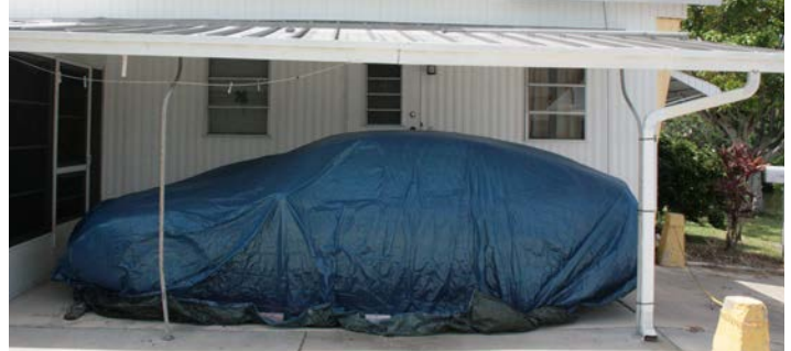
Figure 9. Weak bent post; note sagging roof.
