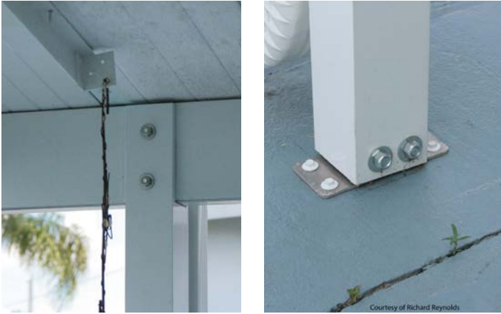
Figure 17. New beam and posts with improved connections supporting old roof.
