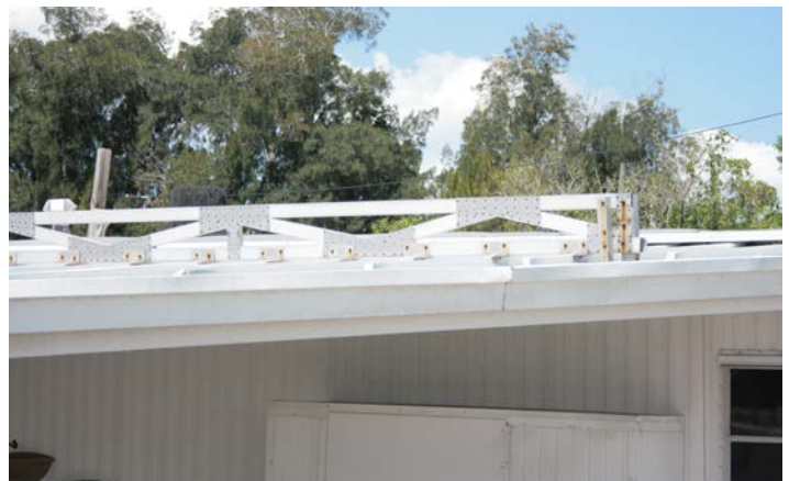
Figure 21a. Truss installed along middle of carport roof to brace pans.
