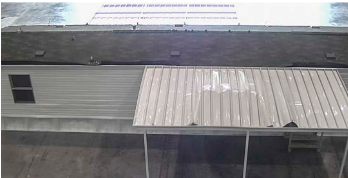
Figure 33. Attachment of roof pans to frame below using #10 TEK screws with combination metal/neoprene washers.
