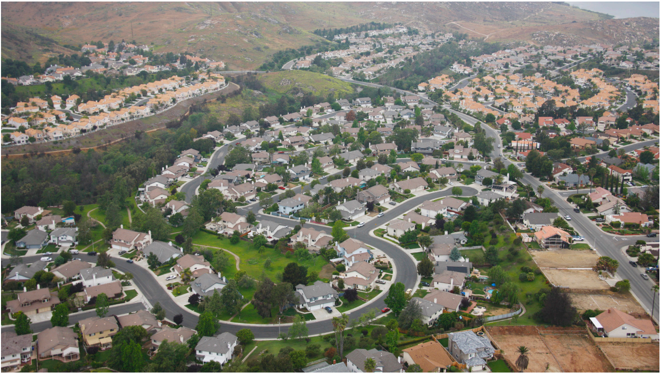
Figure 2: Aerial view of neighborhoods with ongoing new construction after the Southern California Witch Creek Fire in 2007.
