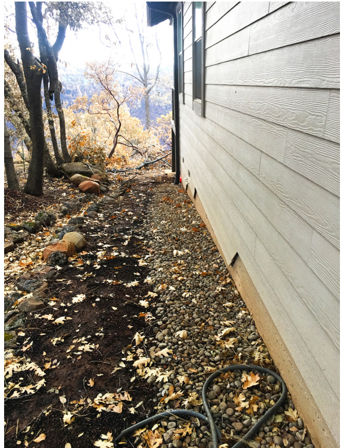
Figure 5: Photograph following the Camp Fire in 2018 showing how the 0-5 foot home ignition zone helped stop the spread of fire to this home. Also note the noncombustible concrete fiber board siding.
