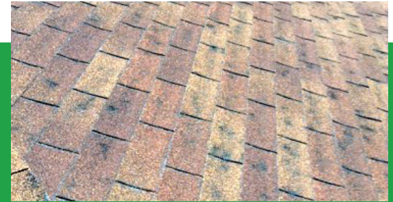
Real hail damage occurs in a random pattern
