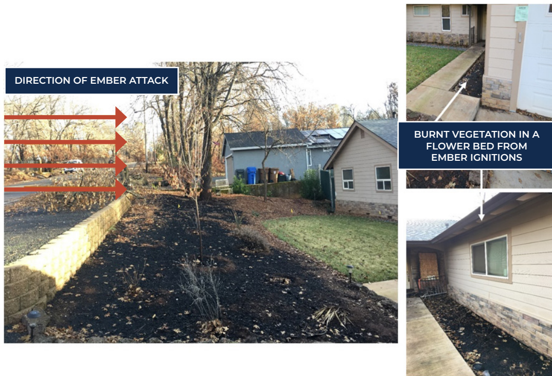
Figure 9. Effectiveness of vegetative fuel management around the house up to property line.
