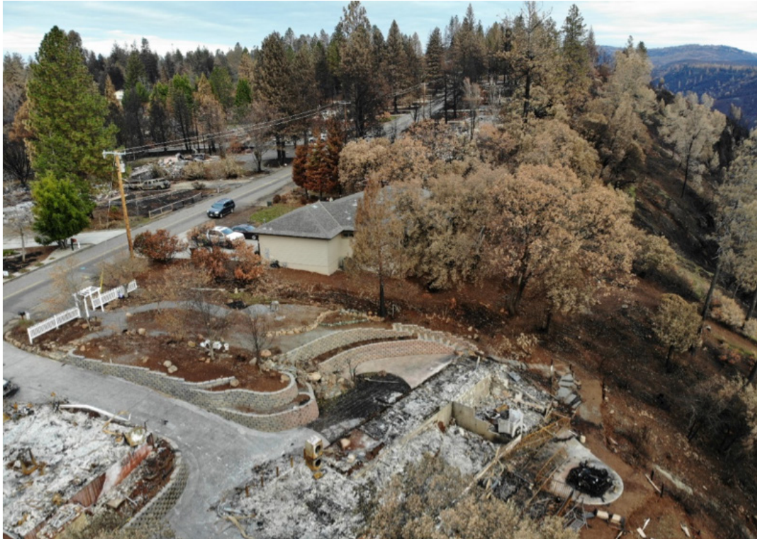
Figure 5. Home on the western edge in the community of Paradise, built after 2008 and to the California Building Code Chapter 7A requirements. Photograph courtesy of Munich Re.
