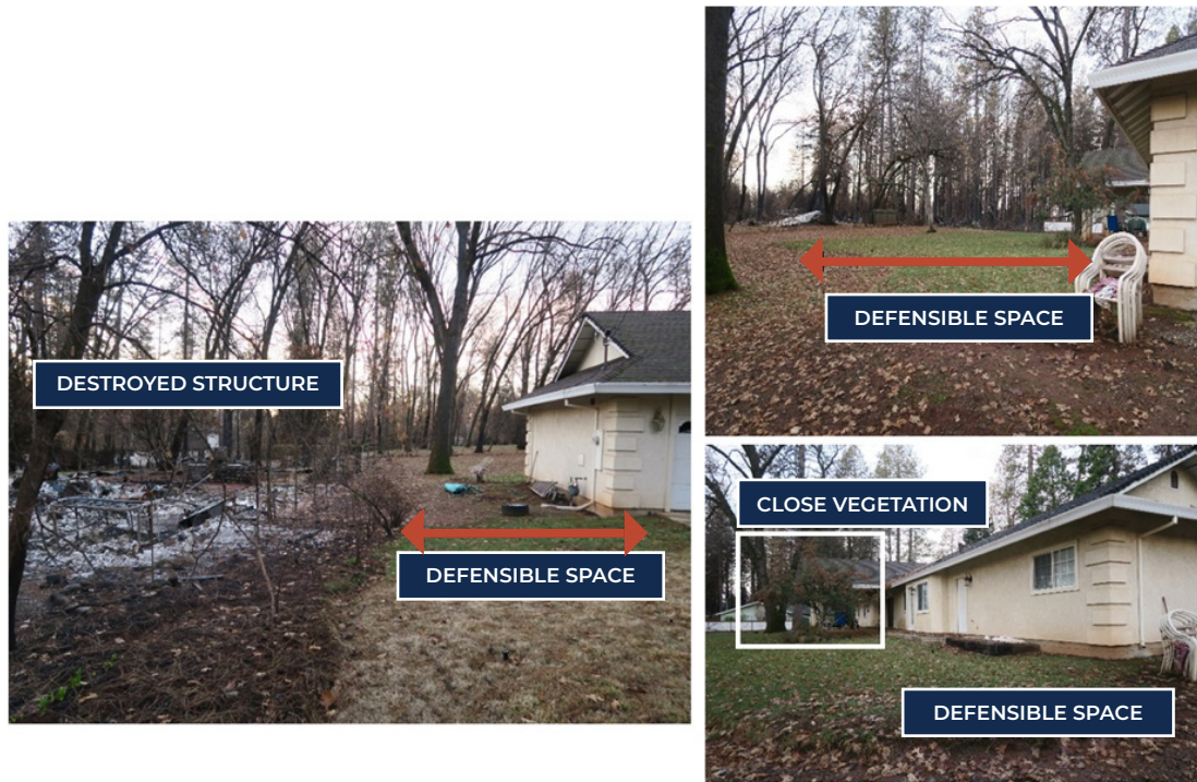
Figure 7. Series of photographs of a home that survived the Camp Fire. The image on the left shows evidence of a nearby structure that was destroyed approximately 20 ft away. The images on the right show in general, well-maintained defensible space except for a tree and large bush near the home (bottom-right image).
