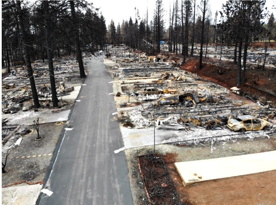
Figure 13. Manufactured-home community completely destroyed in Paradise, California. Separation distance between structures was approximately 10 ft.
