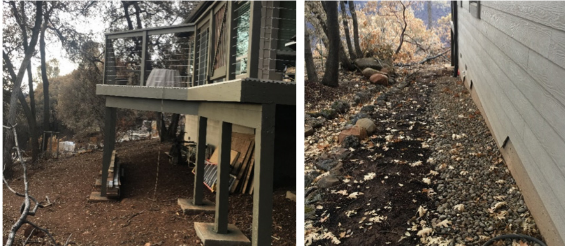
Figure 6. Combination of recommendations and less intense exposure. Well-maintained defensible space and noncombustible zone (rock mulch) around the building and underneath the deck.
