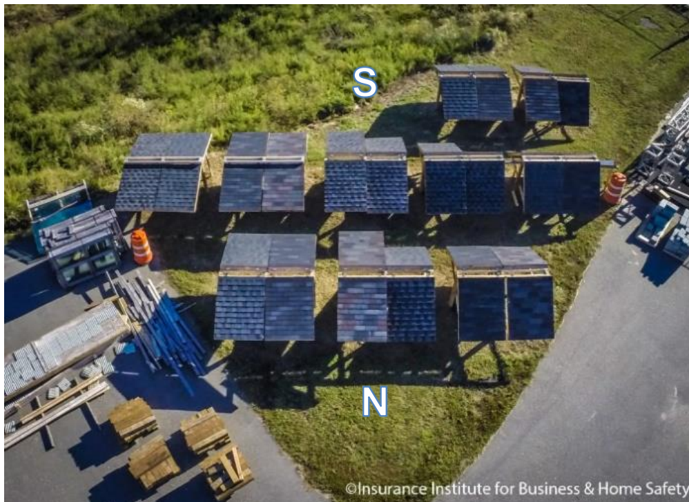
Figure 1. Forty panels (20 pairs) installed at 2:12, 4:12, 6:12, 8:12 and 12:12 pitches.
