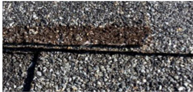
General granule loss common on edges of shingles
