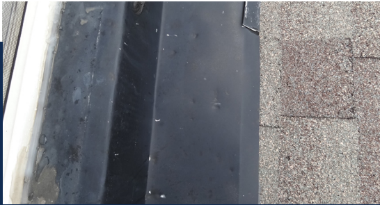
Dents in metal flashing
