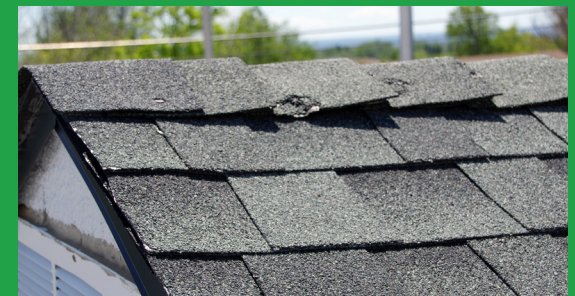
Ridge caps are one of the most hail-vulnerable parts of a shingle roof
