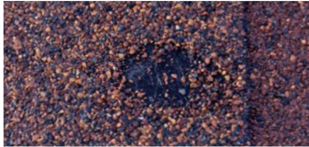
Manufacturer defect that could be mistaken for hail damage
