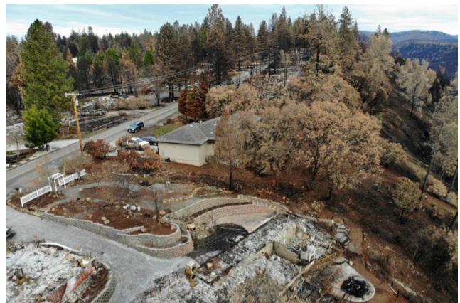
A home on the western edge in the community of Paradise after the Camp Fire. It was built after 2008 and to the California Building Code Chapter 7A requirements. Photograph courtesy of Munich Re.
