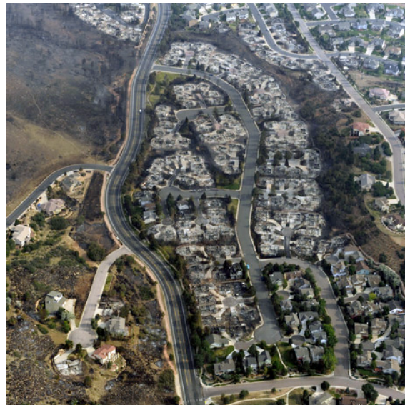
Figure 1. Aerial view of a neighborhood severely damaged during the Waldo Canyon Fire in Colorado in 2008.
