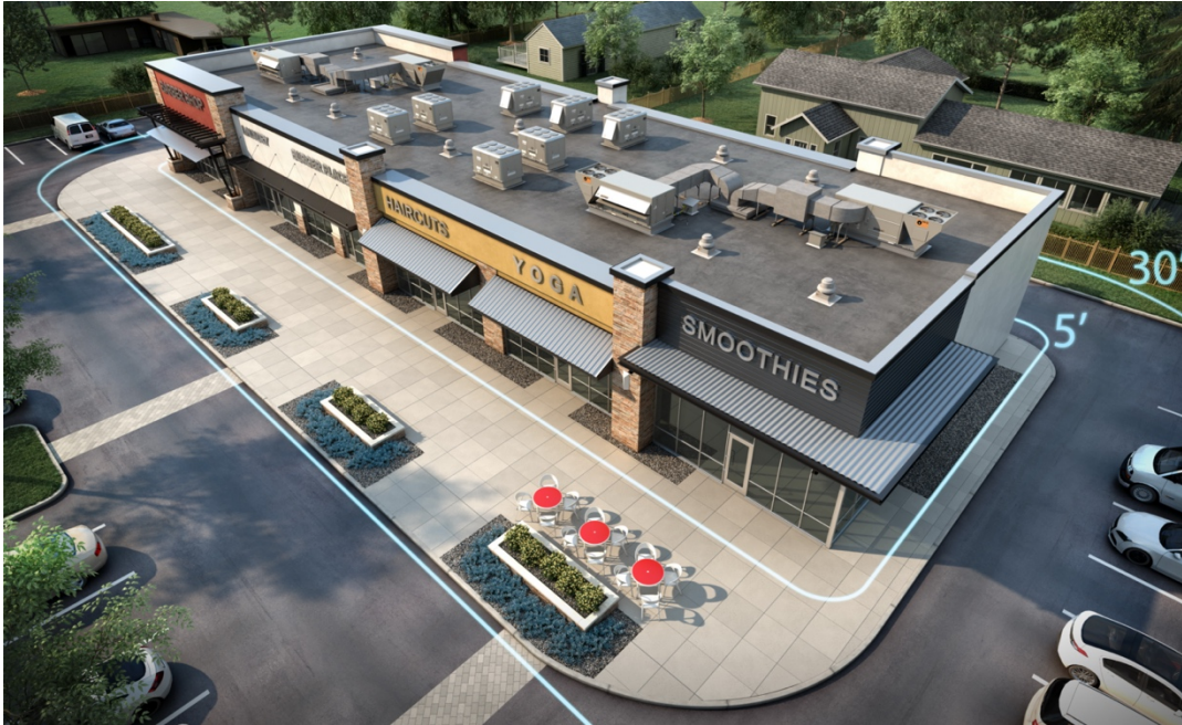
Figure 3. Aerial view of a typical suburban strip mall highlighting the 0–5 ft noncombustible zone.
