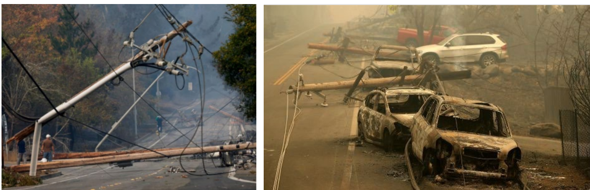
Figure 12: Electrical utility infrastructure that fell in the roadways in Paradise, CA during the Camp Fire in 2018, hindering the evacuation of residents from the Town of Paradise. Photographs courtesy of CAL FIRE.
