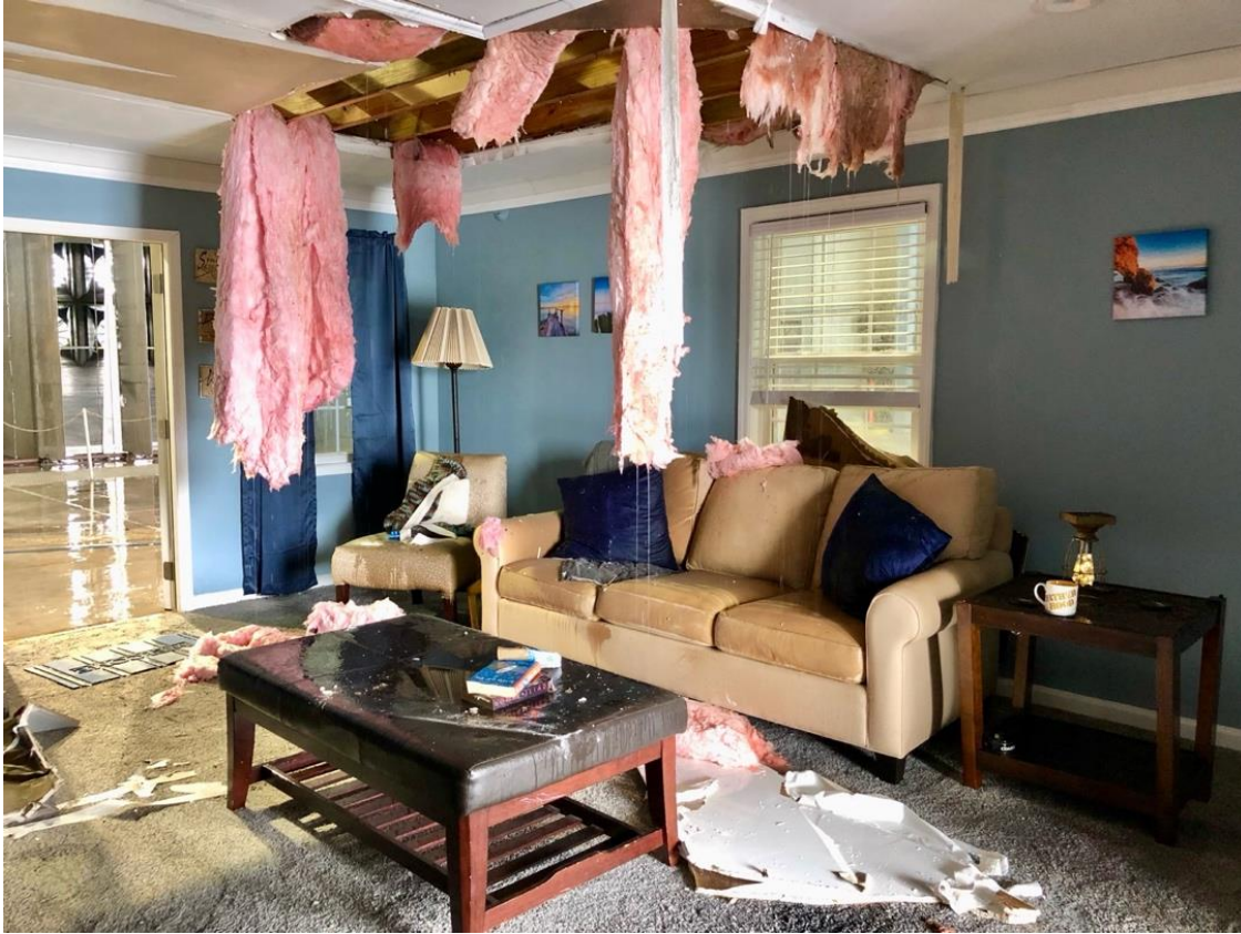
Figure 3. Photograph of interior water intrusion damage following a full-scale wind-driven rain simulation in 2019 at the IBHS Research Center.
