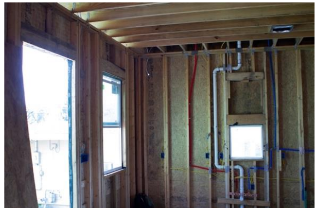
Figure 6. Plumbing in exterior walls of a home under construction in Louisiana.
