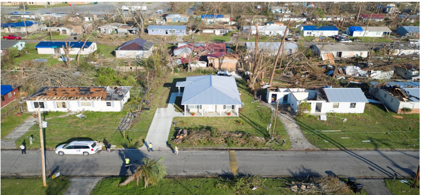
Figure 1: Photograph of a Habitat Strong house (center) following Hurricane Michael (2018) in Panama City, Florida. This home was built to FORTIFIED Gold™ by Habitat for Humanity. It suffered only minor siding damage and likely experienced peak gust wind speeds of 140–150 mph.
