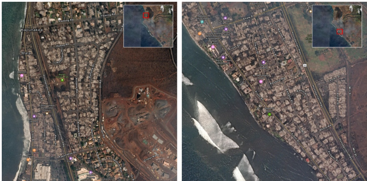
Figure 2: Satellite imagery of two areas where some of the most intense fire exposure possibly occurred, (left) south of Fleming Rd. to Kapunakea St. and (right) the area south of Shaw Street and bounded on the east side by the Honoapiilani Highway, including along Front Street. Satellite imagery courtesy of Maxar.
