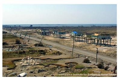
Figure 3: Homes on the Bolivar Peninsula following Hurricane Ike (2008). These structures were elevated above the 100-year flood level and built to the IBHS Fortified standard.
