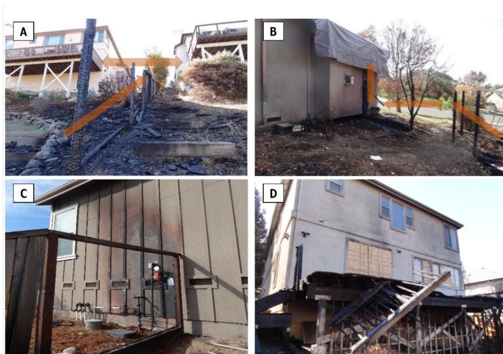
Figure 9: Examples of structural fuel connectivity and the role in damaging the main building in a parcel during the Glass Fire. A combustibile fence (A and B) supported flaming ignition, moving from downhill all the way to the main building, and caused severe damage (C and D). A and B are annotated with arrows representing the estimated direction of fire spread.
