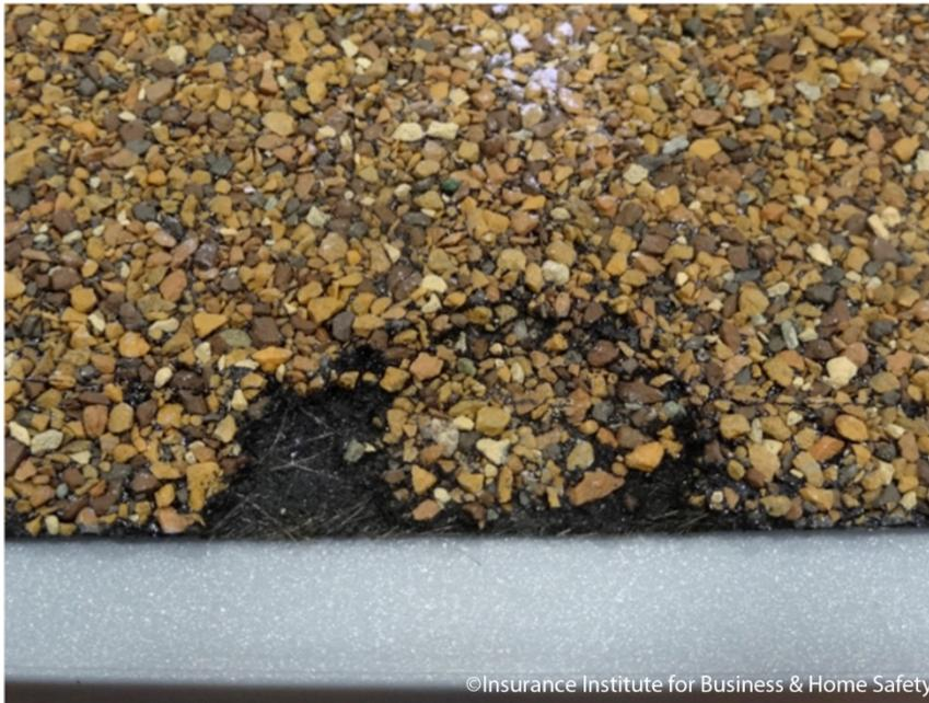
**Figure 3.18.2.1-1.** Example photograph of patch granule loss.
