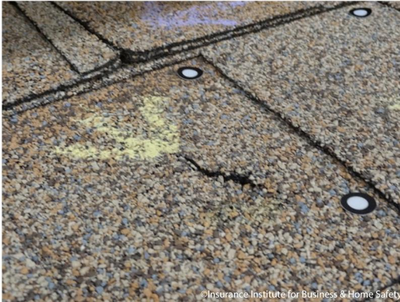
**Figure 3.18.3-1.** Example photograph of breach.
